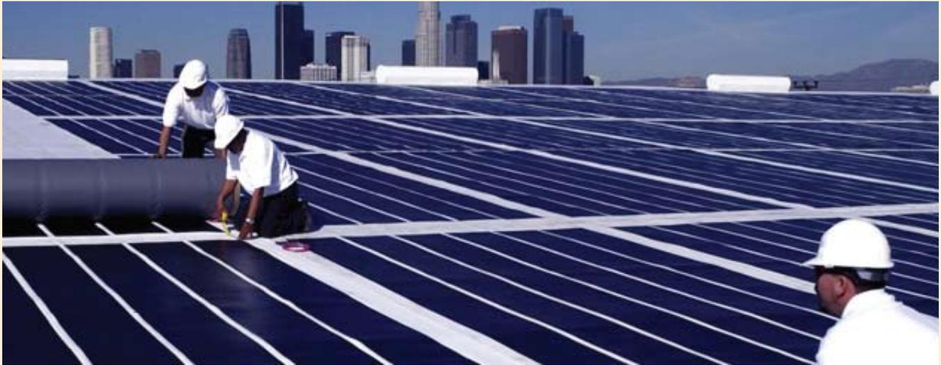
Uni-Solar's Flexible Thin Film Solar Panels
